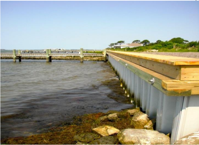
Bulkhead or Seawall
